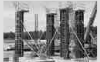
Column Formwork
